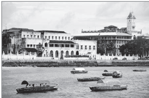
Figure 13. Palace Museum and House of Wonders, the former ceremonial palace for Sultan barghash, Stone Town, Zanzibar. Photo by Michael King.
